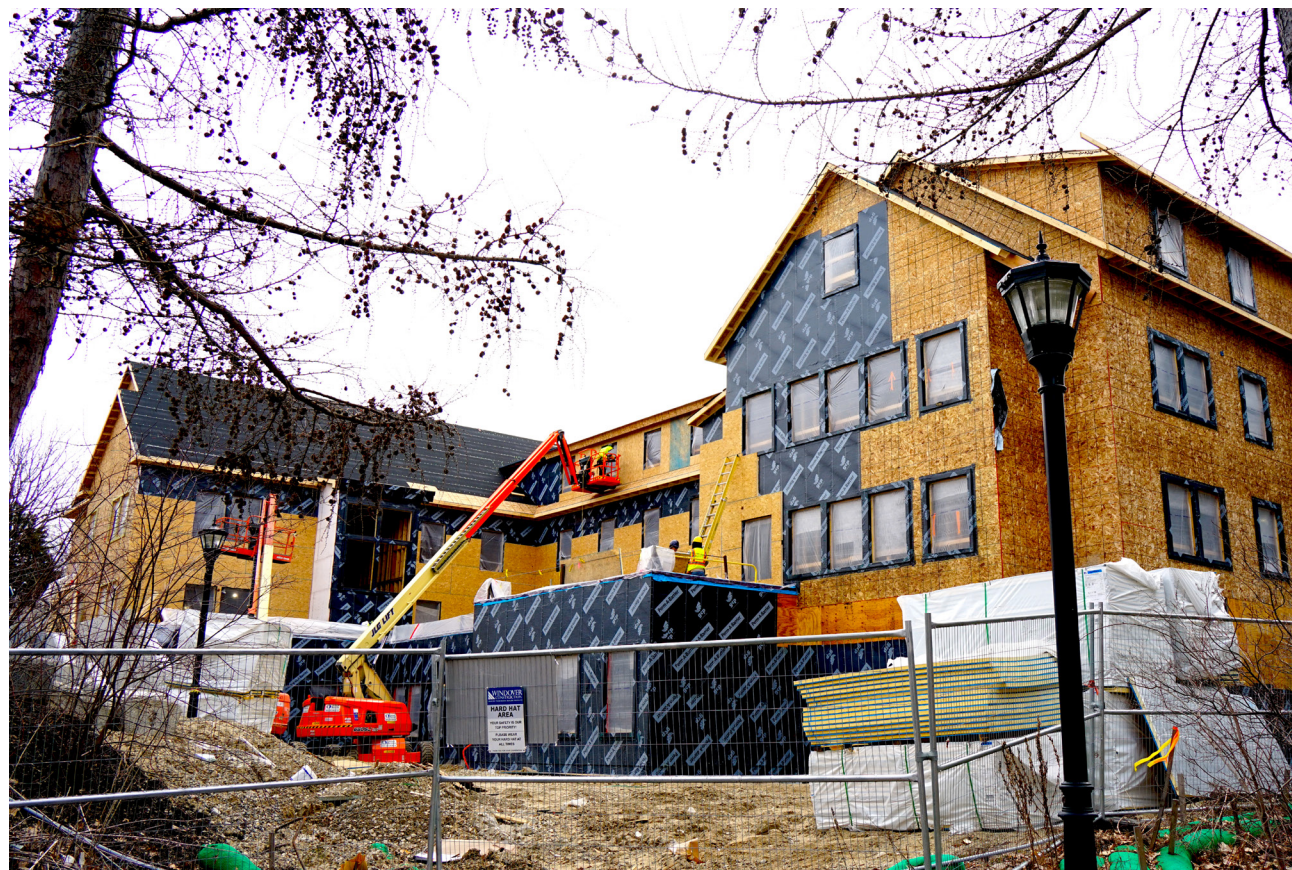
Front Street Commons continues construction.
