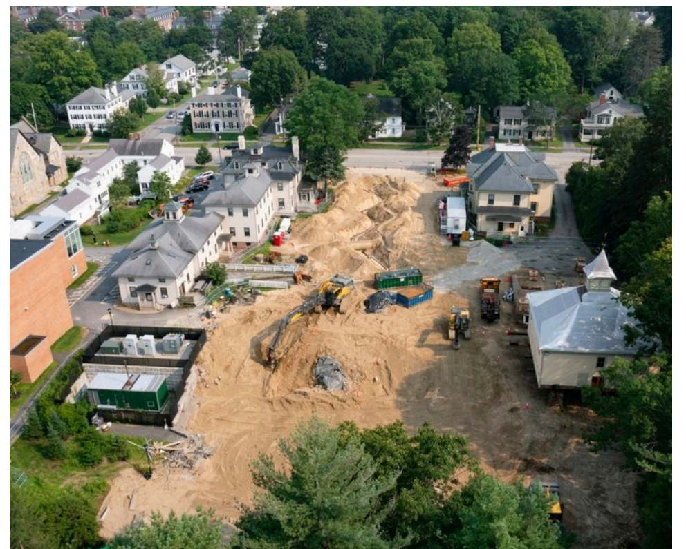
Front Street Commons under construction.
